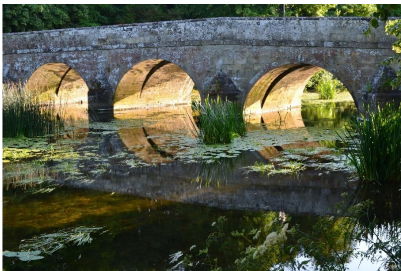
Figure 24 View of Blandford Bridge
